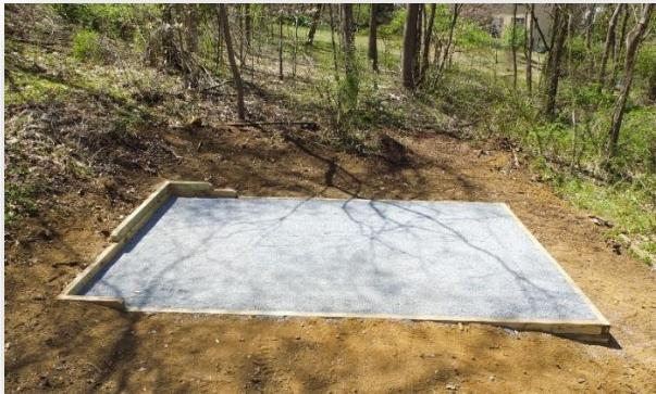
A **4-inch slab** (min) is generally a good thickness for a typical shed. This type of concrete floor can be poured in most locales on a **4-inch base of compacted gravel**.
